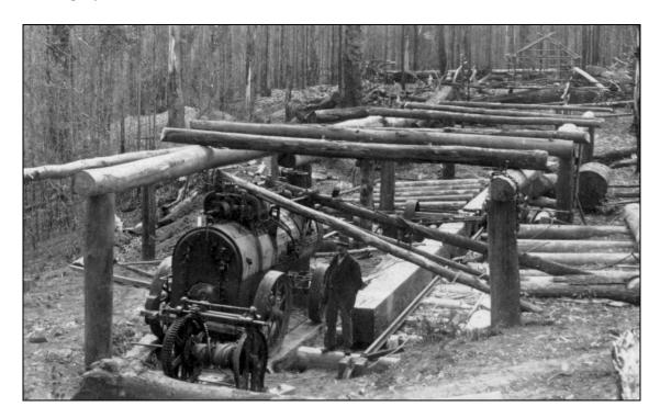
The photograph above (*Hayden's mill under construction in the Otways in 1919*) shows almost every facet of modern mill construction which will be typical of the majority of the sites to be visited during the present survey (*Author's collection*).
